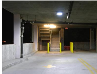
FIGURE 2. LED SYSTEM AT FULL OUTPUT 82.5W 6.9 FC WITH 3:1 UNIFORMITY
